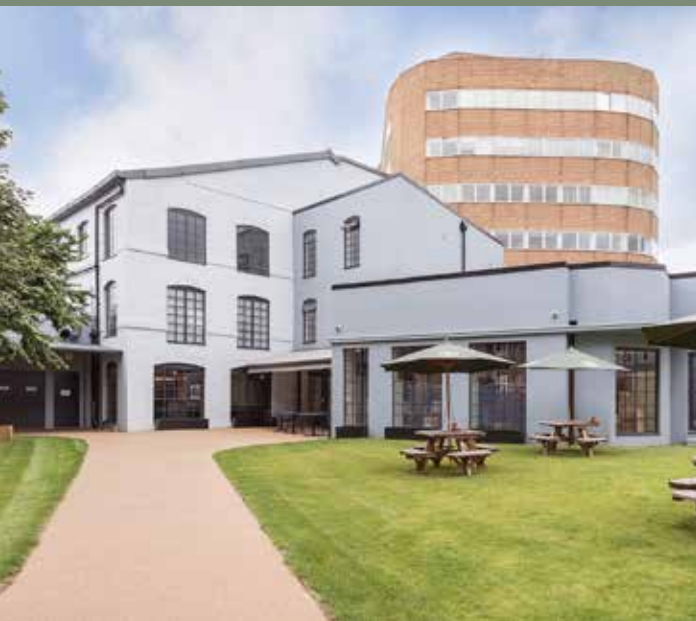
212 New Kings Road SW6 4NZ
