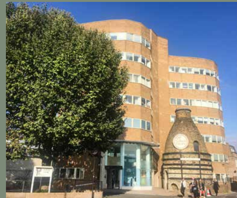
210 New Kings Road SW6 4NZ
