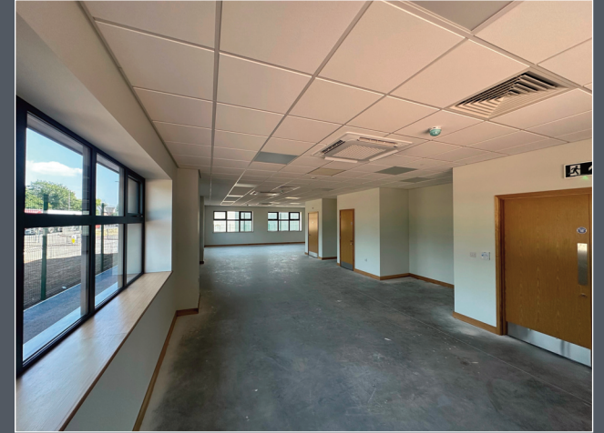
Ground Floor Office
