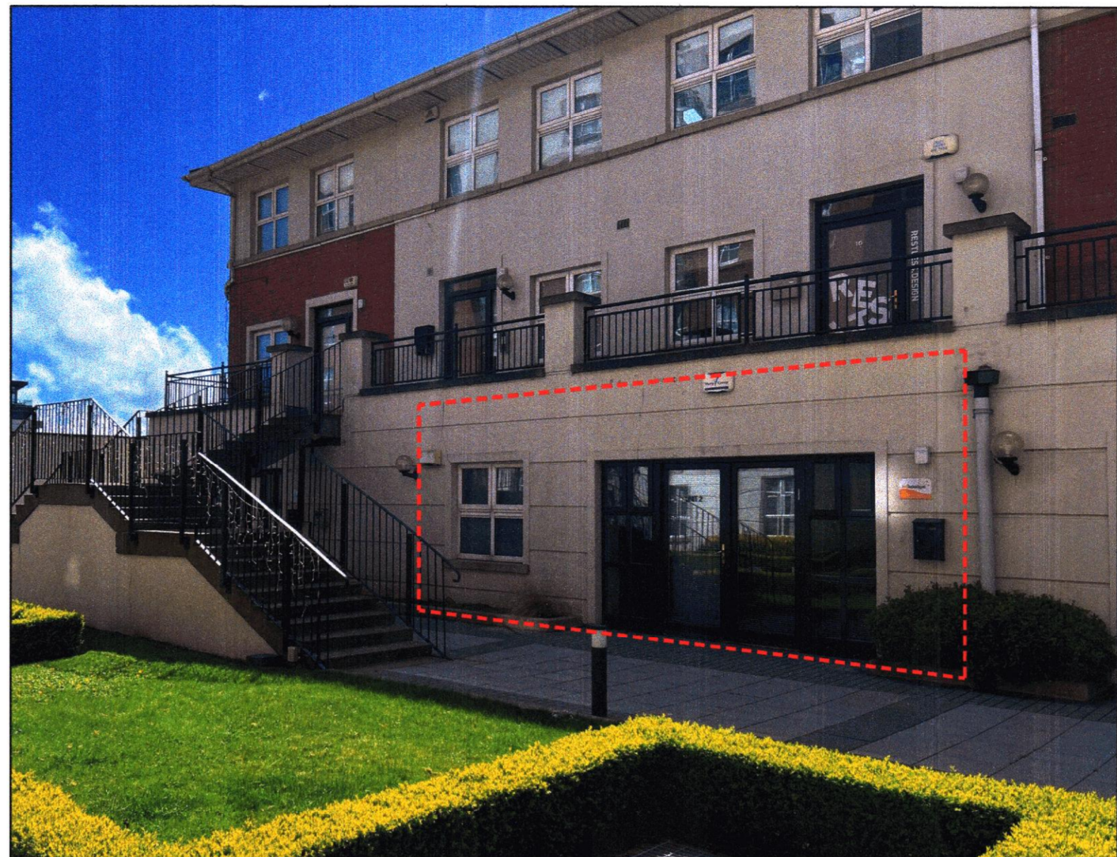
PHOTO OF EXISTING NORTH ELEVATION NO ALTERATIONS REQUIRED NOT TO SCALE
