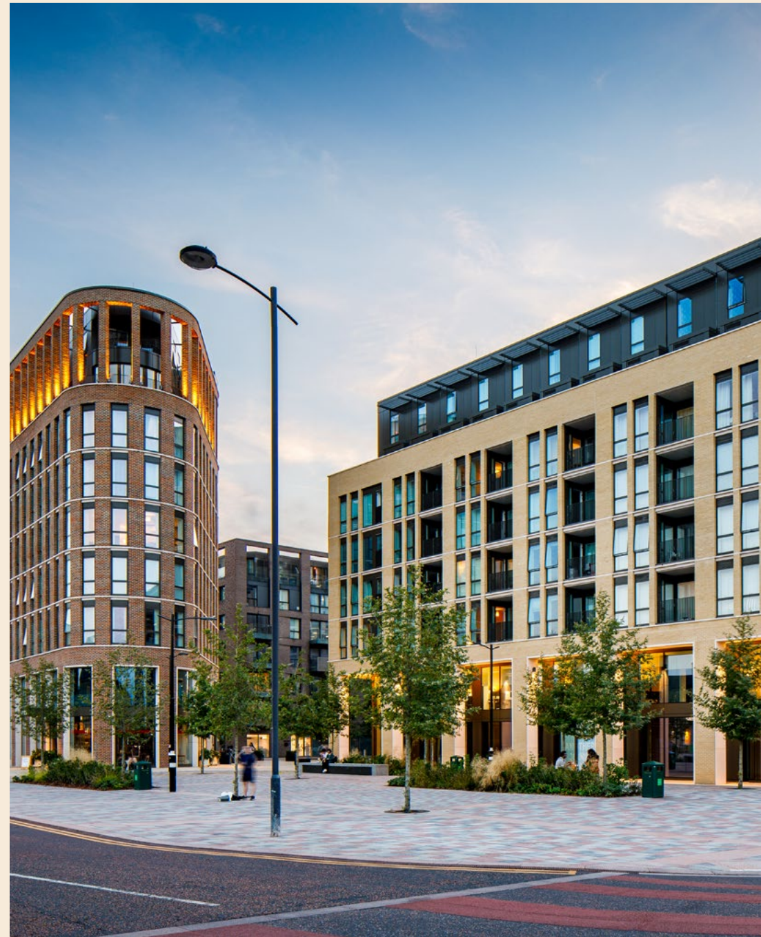
Frontage of 3 & 4 Station Square
