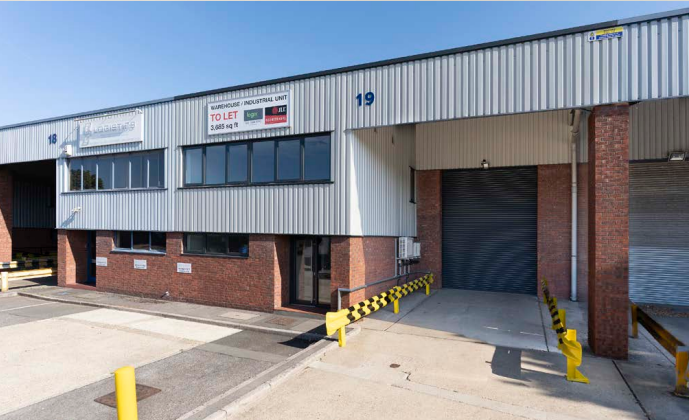
Refurbished warehouse example (Unit 19)
