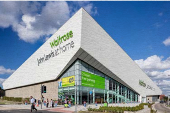
A 110,000 sq ft combined Waitrose and John Lewis at Home store was completed in 2015.
