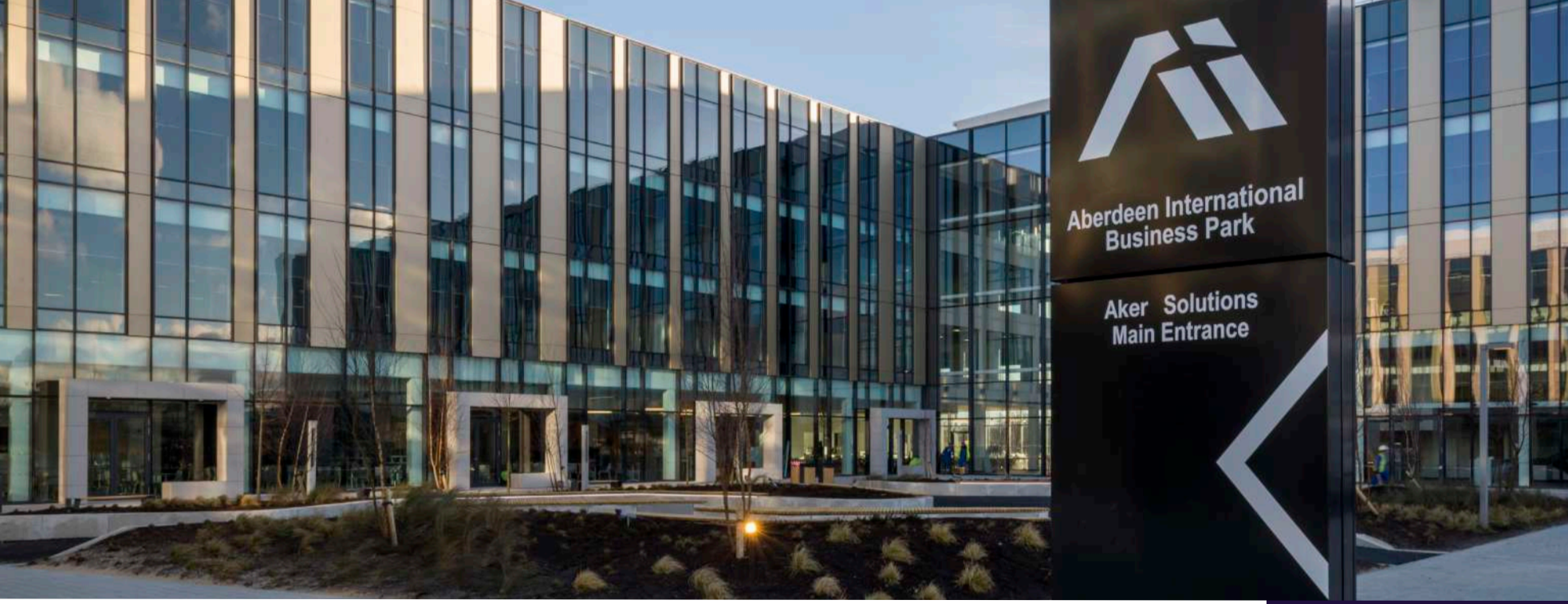
Aberdeen International Business Park (AIBP)
