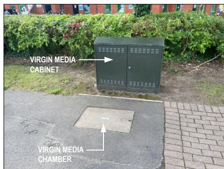
PHOTOGRAPH 5 EXISTING VIRGIN MEDIA CABINET AND CHAMBER IN FOOTWAY ON MAIN AVENUE ADJACENT TO BUILDING
