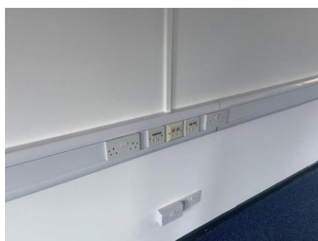
PHOTOGRAPH 11 TYPICAL VIEW OF SURFACE TRUNKING AFFORDING ACCESS FROM CEILING FOR INTERNAL TELECOMS CABLING
