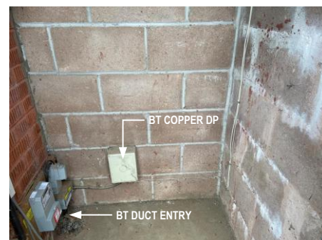
PHOTOGRAPH 9 TYPICAL VIEW OF BT DUCT ENTRY POINT AND BT COPPER SERVICES/ DISTRIBUTION POINT
