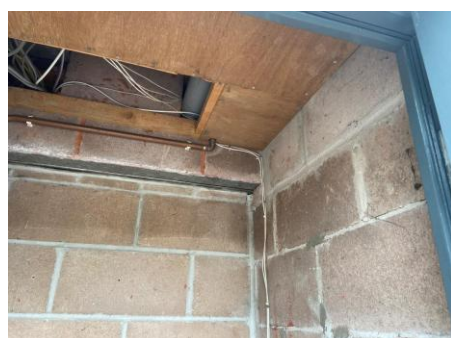
PHOTOGRAPH 10 TYPICAL VIEW OF BT COPPER SERVICES EXITING THE REAR SERVICE CUPBOARD INTO SUSPENDED CEILING
