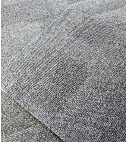
Existing carpet tiles relaid.
