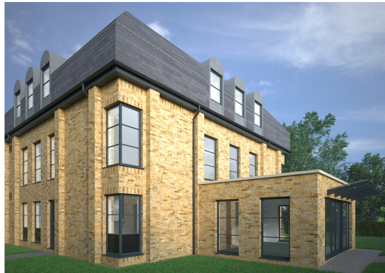
Stoneham Place post refurbishment
