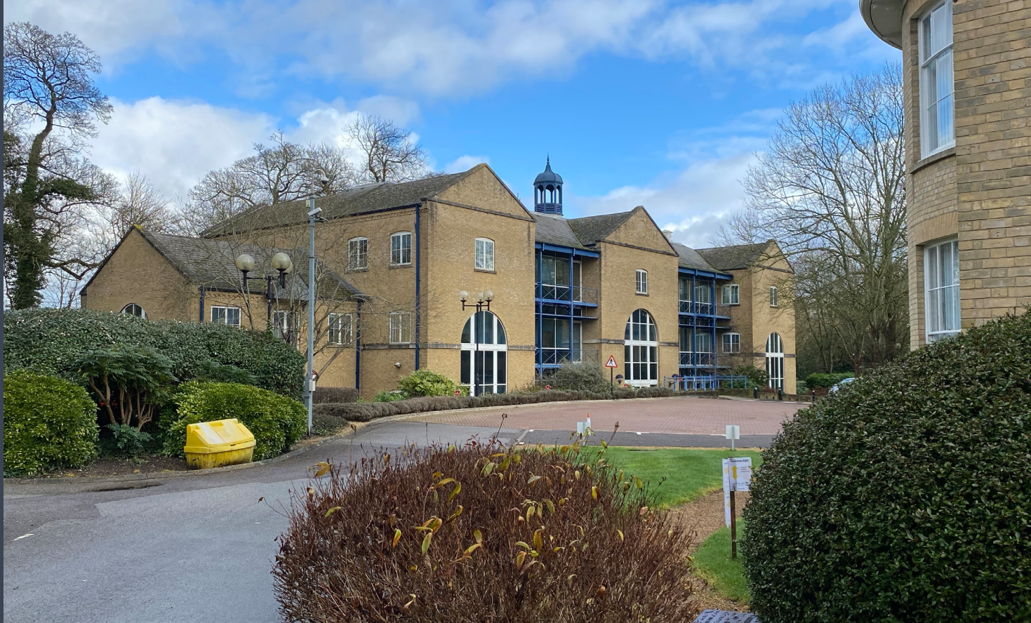
Stoneham Gate (before refurbishment)
