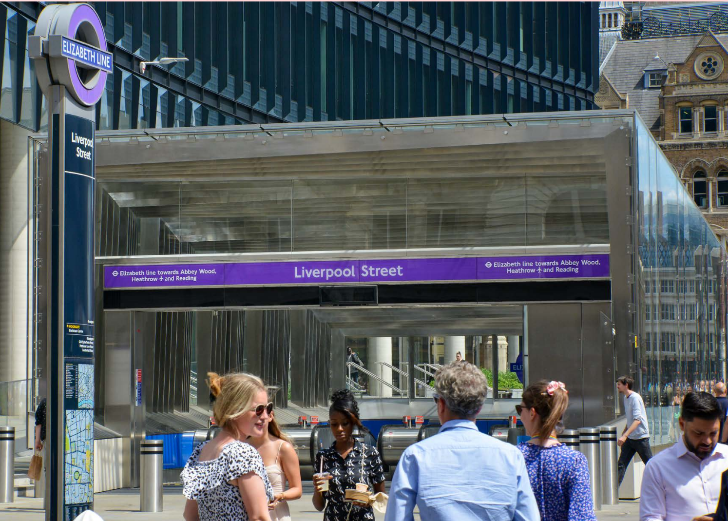
ELIZABETH LINE ENTRANCE - LIVERPOOL STREET STATION
