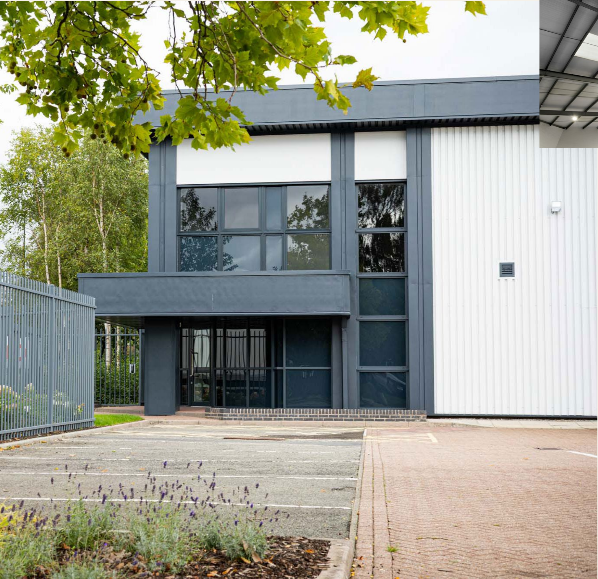
● Unit A Exterior
