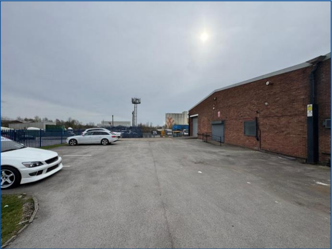
Yard and loading area
