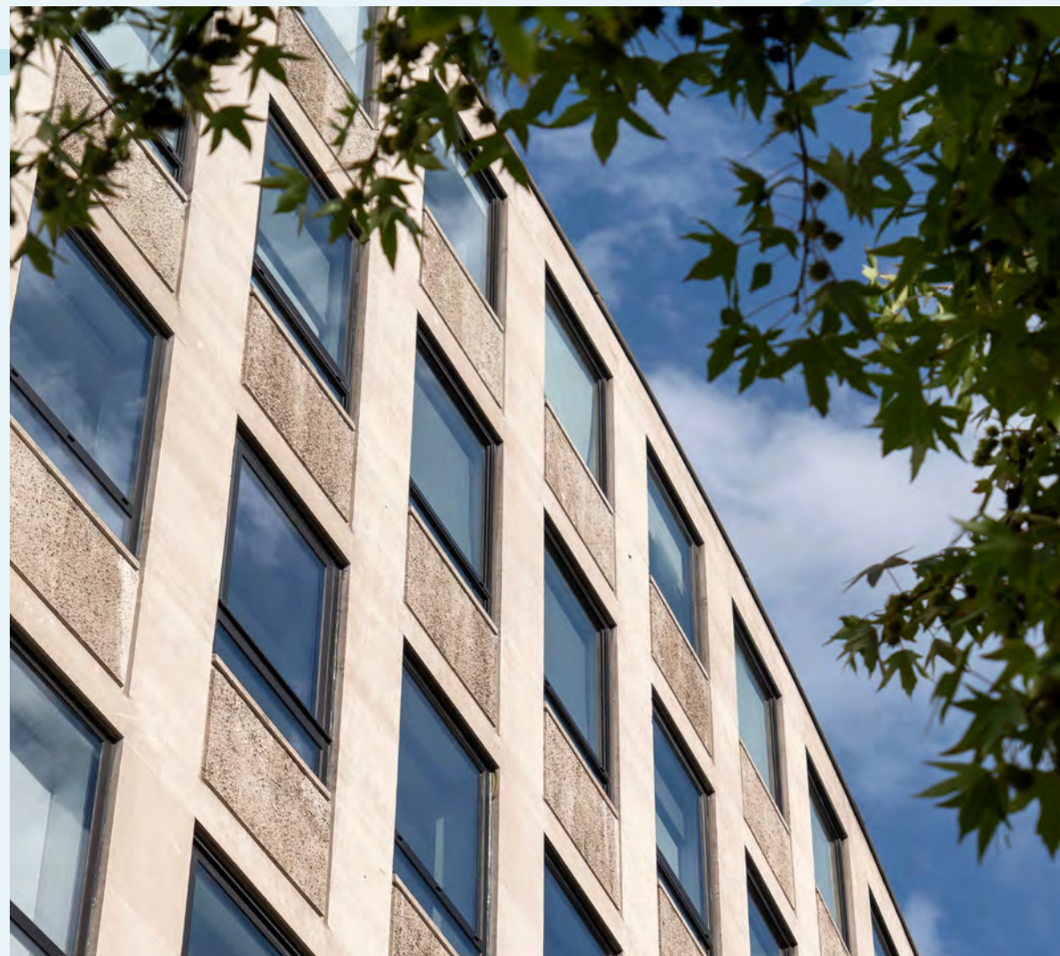
Building façade detail facing Cheapside
