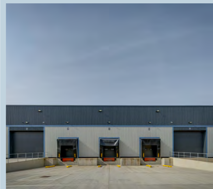
3 dock level doors & 3 level access doors
