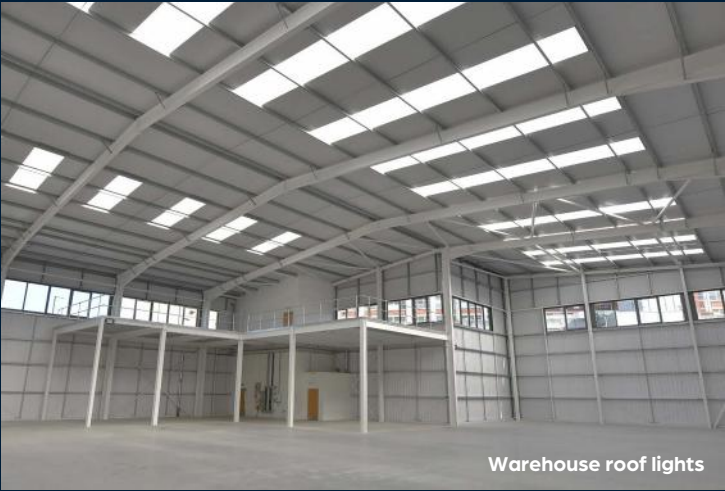
15% warehouse roof lights increasing natural lighting
