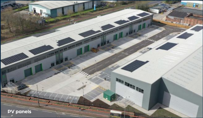
Warehouse roof lights
