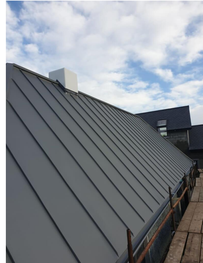
Dark grey zinc for feature roof to apartments
