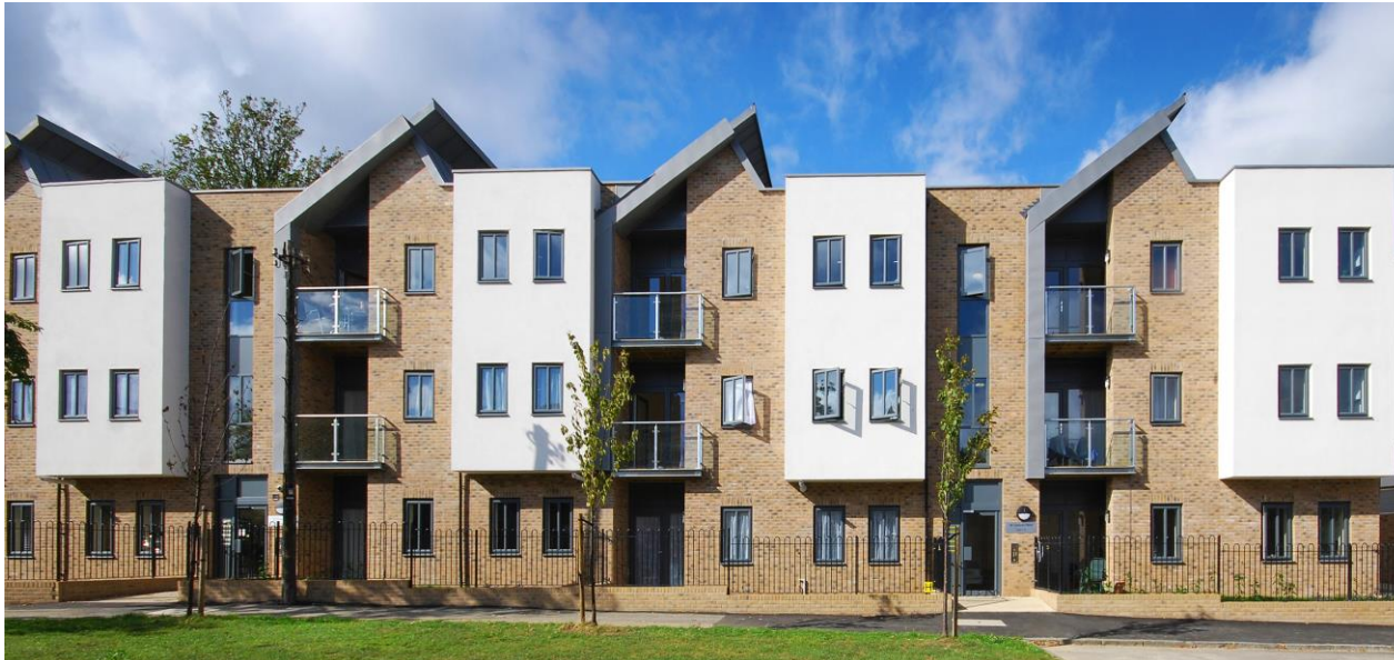
Castledine Road, London – new build Residential / Mixed use Development
