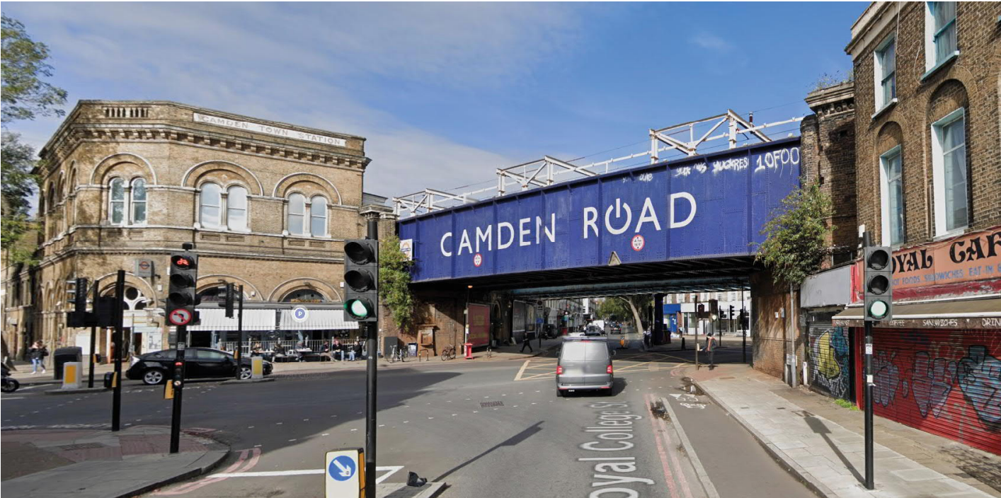
Fig 05: Camden Road Station
