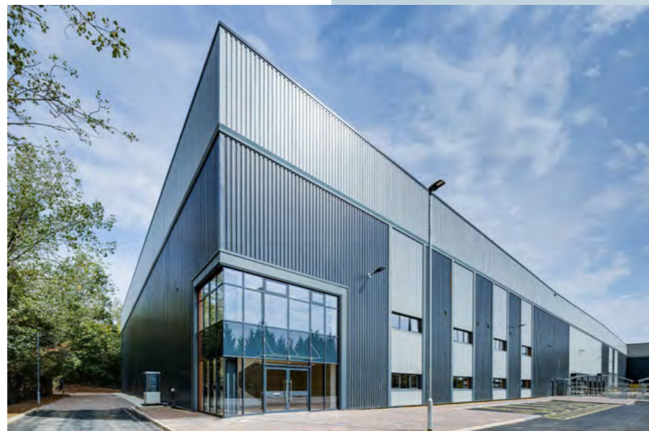
Reception entrance & EV charging unit
