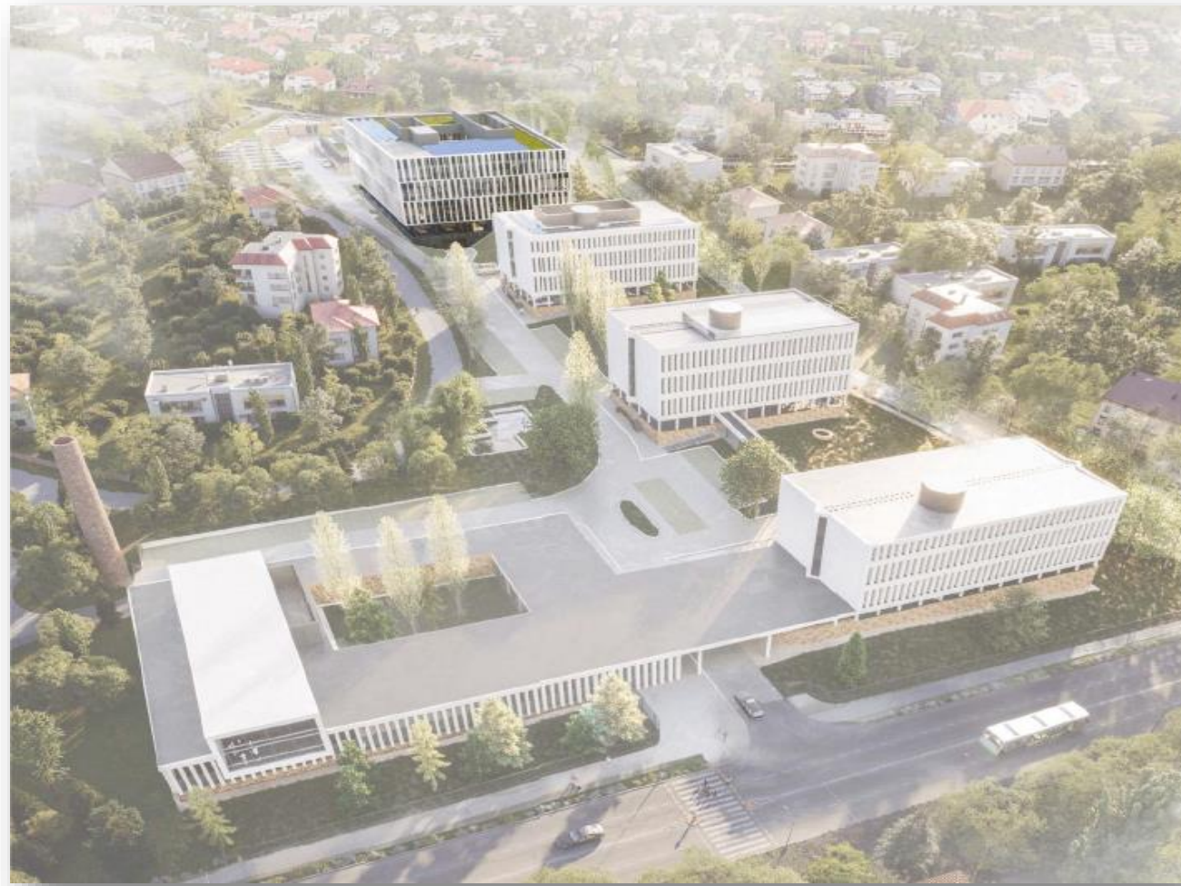
Pusztaszeri Office Park GLA: 16,500 sq m Status: Under refurbishment Location: Buda Hills
