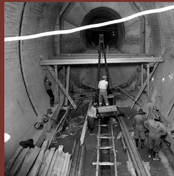
1954 Constructed to serve as Manchester's telephone exchange
