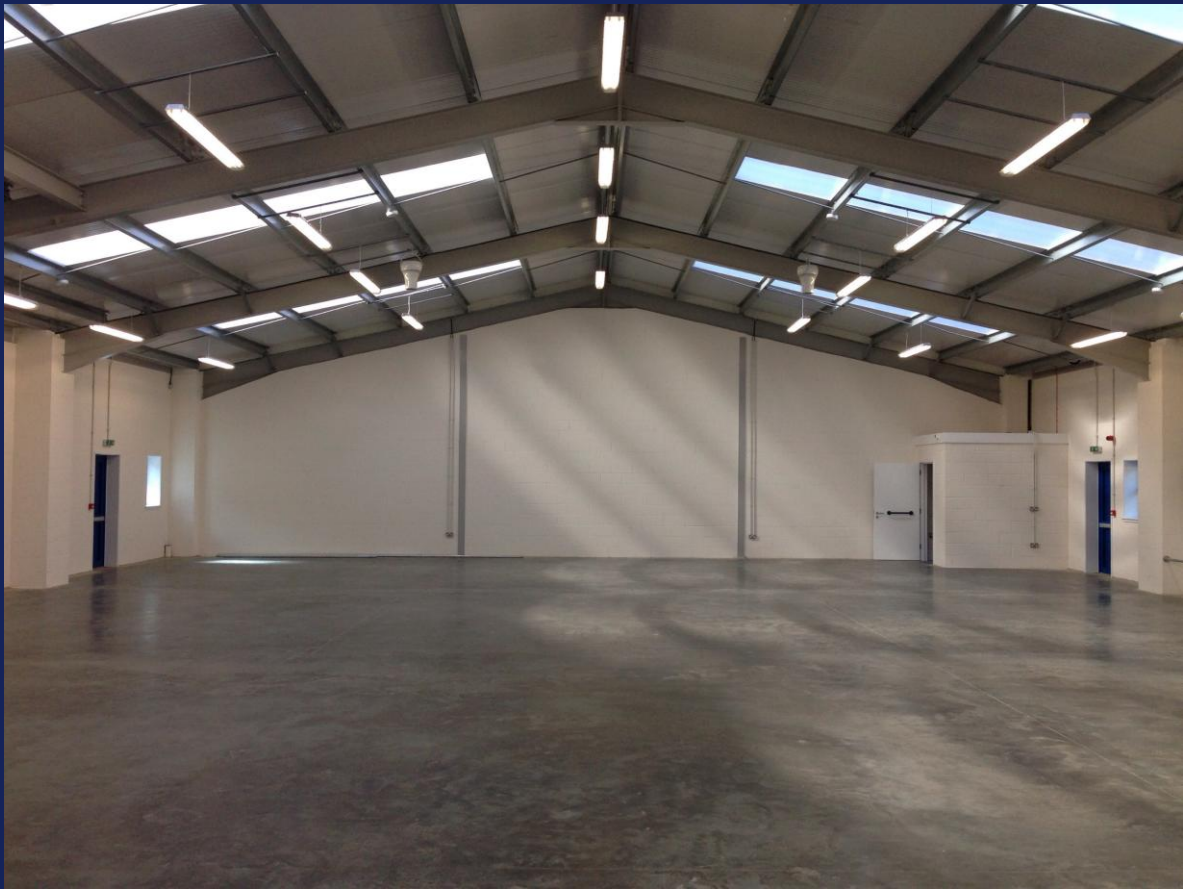
Warehouse prior to occupation
