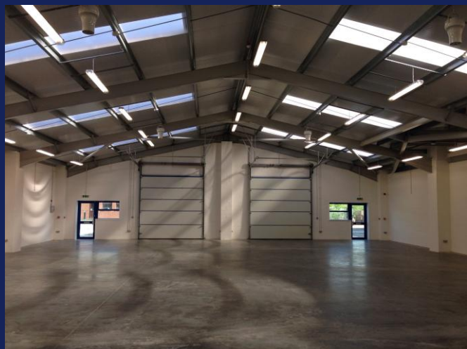
Warehouse prior to occupation
