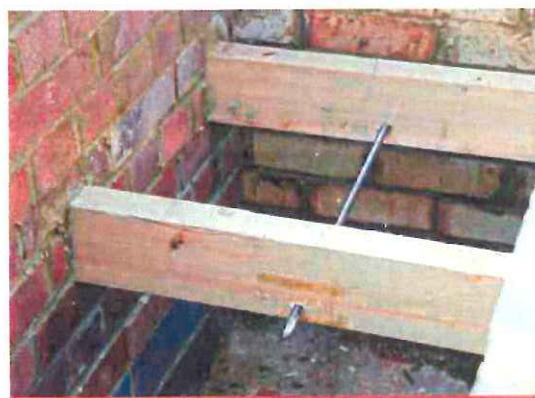
BowTie HDs installed through parallel floor joists
