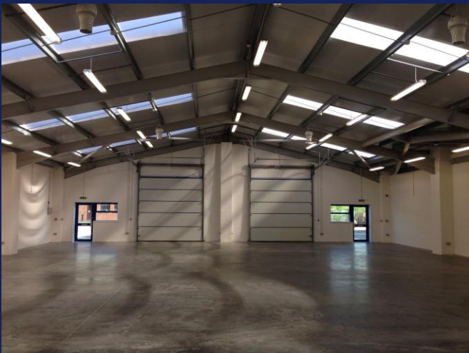
Warehouse prior to occupation
