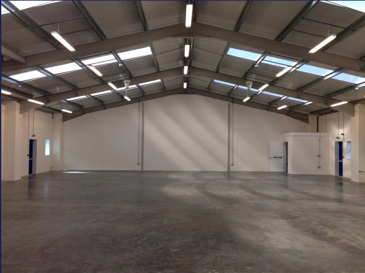
Warehouse prior to occupation
