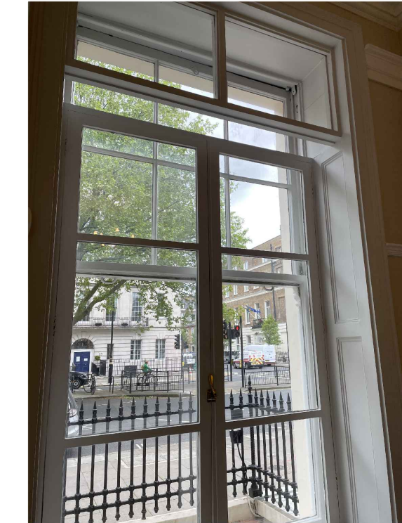
EXISTING SECONDARY GLAZING TO GRD FLOOR
