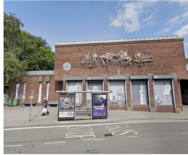
VIEW FROM BETHLEHEM STREET
