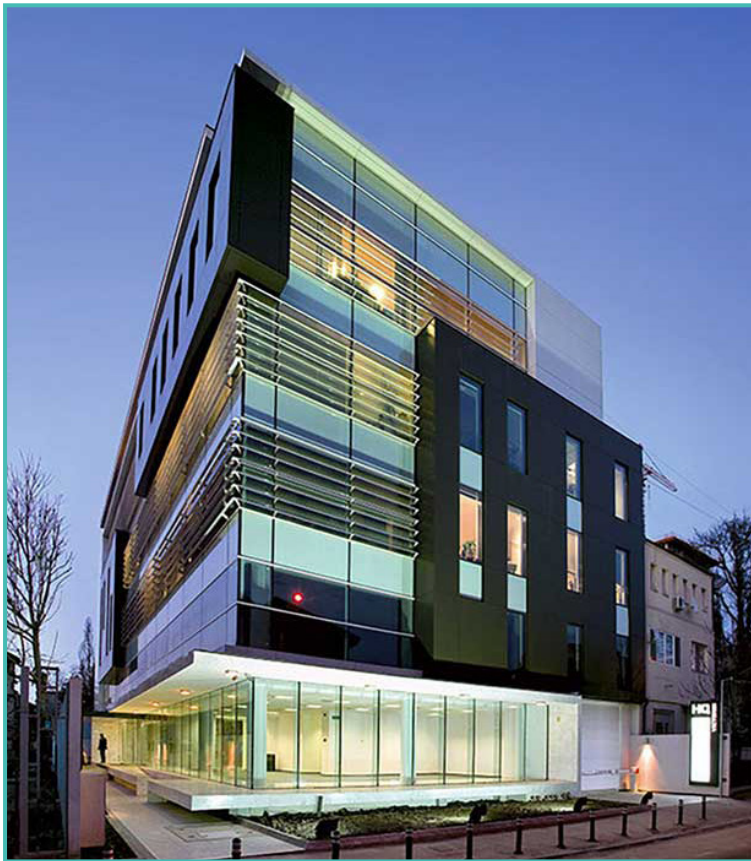
HQ Victoriei, 8.900 sqm office building is located in the most prestigious business district of Bucharest, around Victoriei Square. Grigore Alexandrescu 59, Bucharest, Romania
