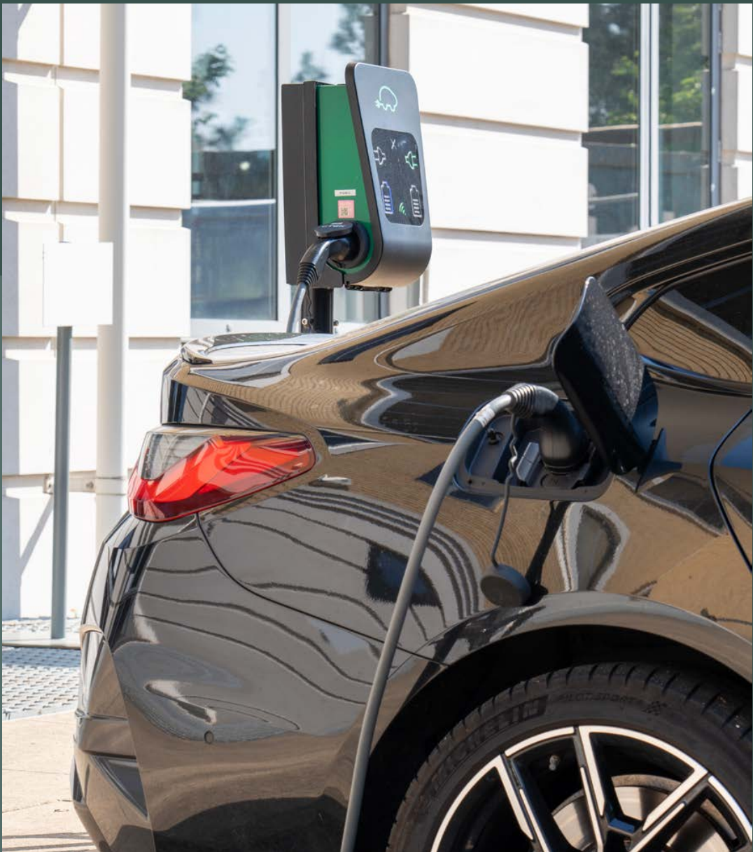
EV charging point
