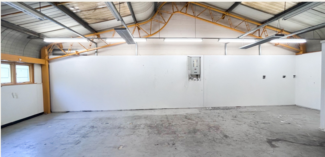
Unit 3 (Upper Floor on Oppidans Road)
