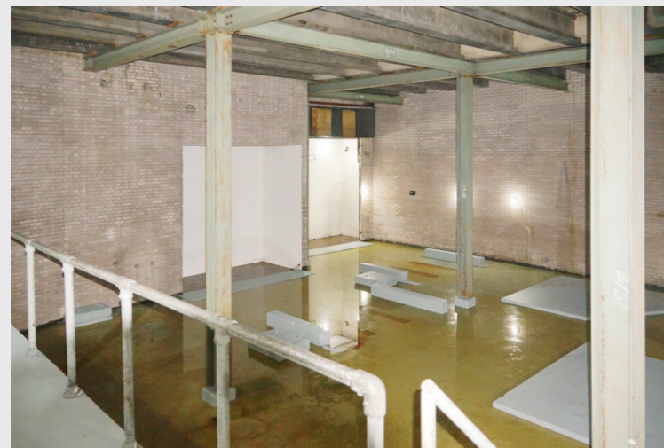
➤ View towards double height space
