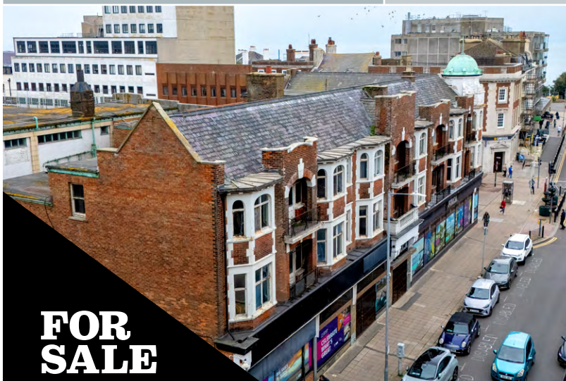
THE PROPERTY, SOUTH WEST VIEW
