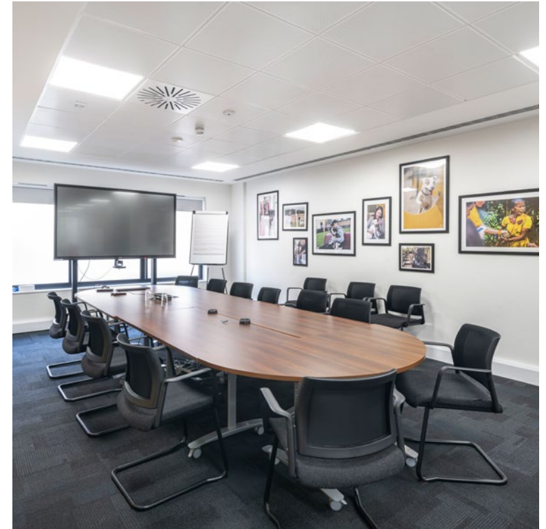
Metal tile ceilings with plasterboard margins
