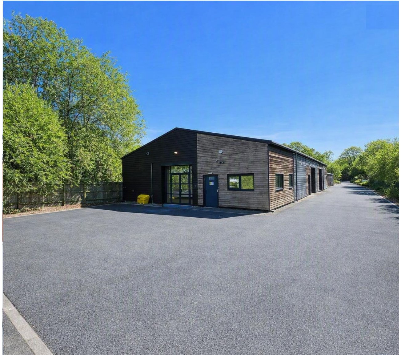
Unit 1, The Sidings, Station Works, Claverdon, CV35 8PE
