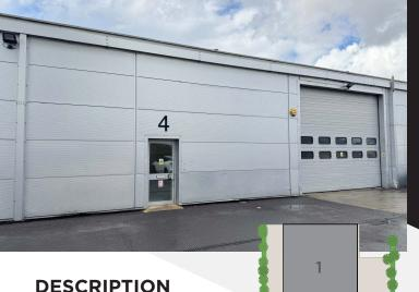
Unit 4 is a mid-terrace unit of steel portal frame construction with metal cladding under a dual pitched roof. The unit is to undergo a refurbishment to provide clear span warehouse space benefitting from a roller shutter door, 5.15m eaves and 3 phase power. Generous parking and loading facilities.
