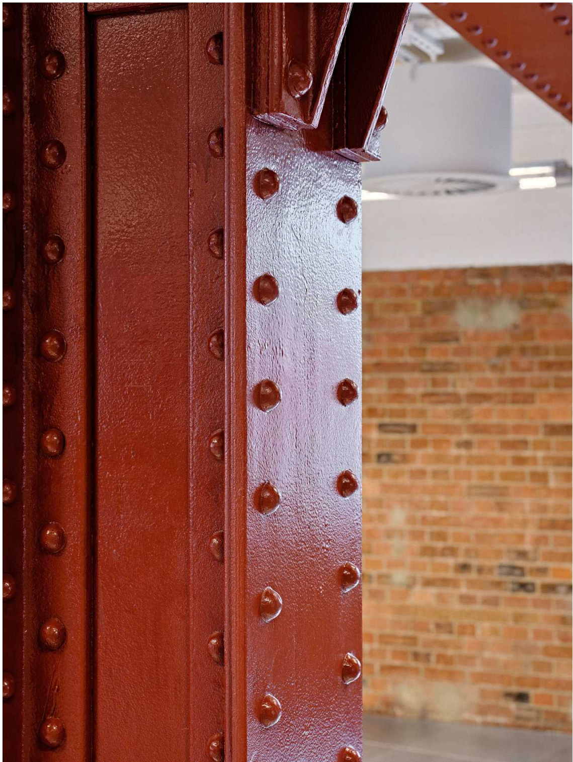
Retained steel columns
