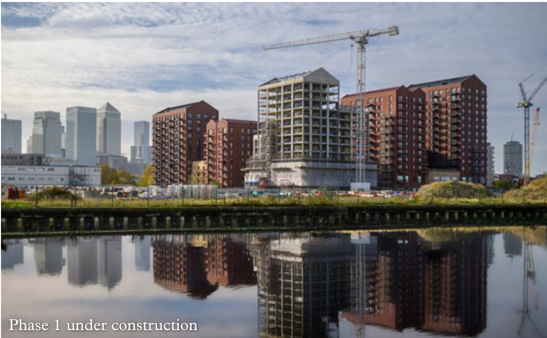
Phase 1 under construction
