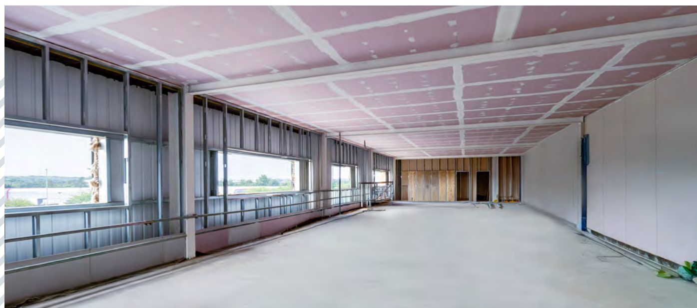
First Floor Office Space
