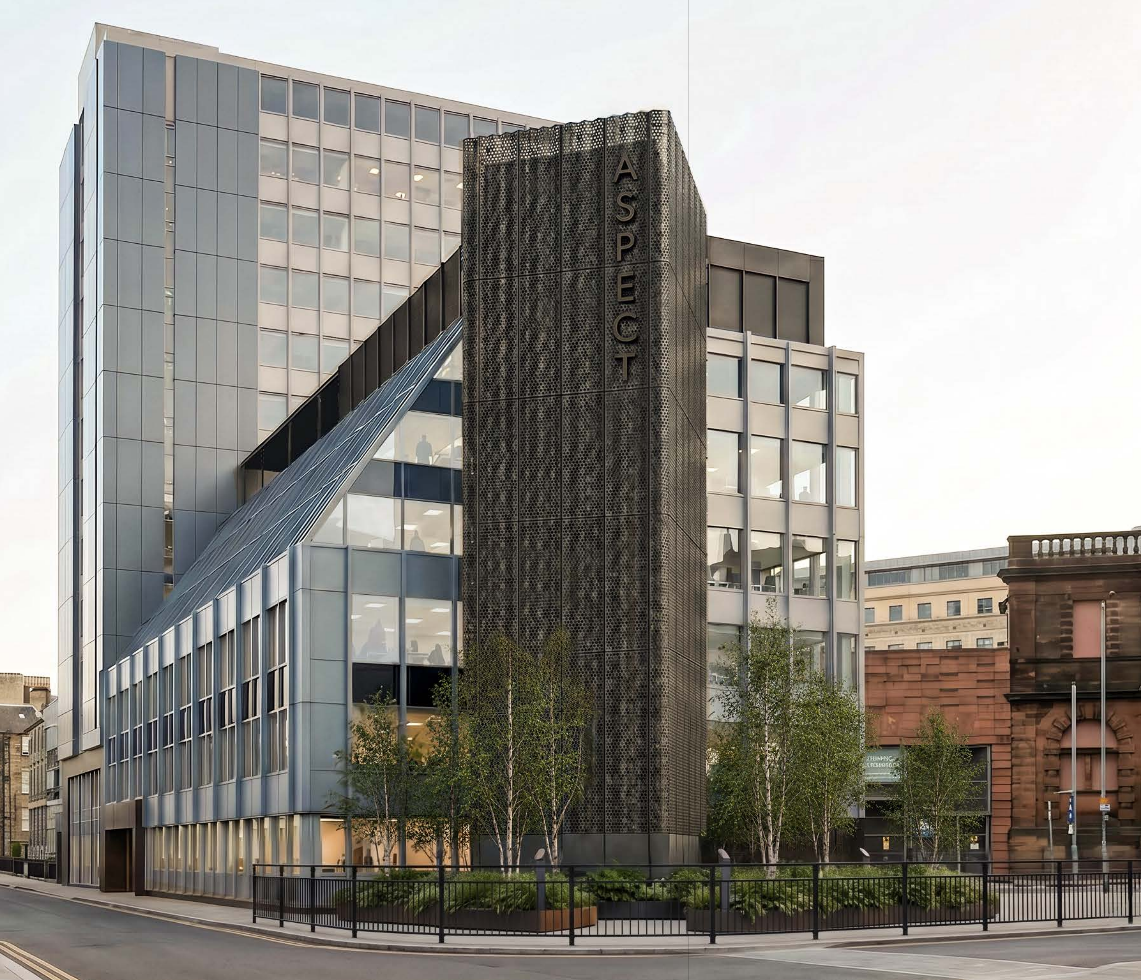
◀ View of The Aspect Building on the approach from Haymarket Station
