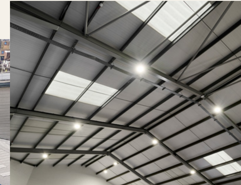
• Newly fitted roof panels for enhanced natural lighting increasing staff welfare and efficiency
