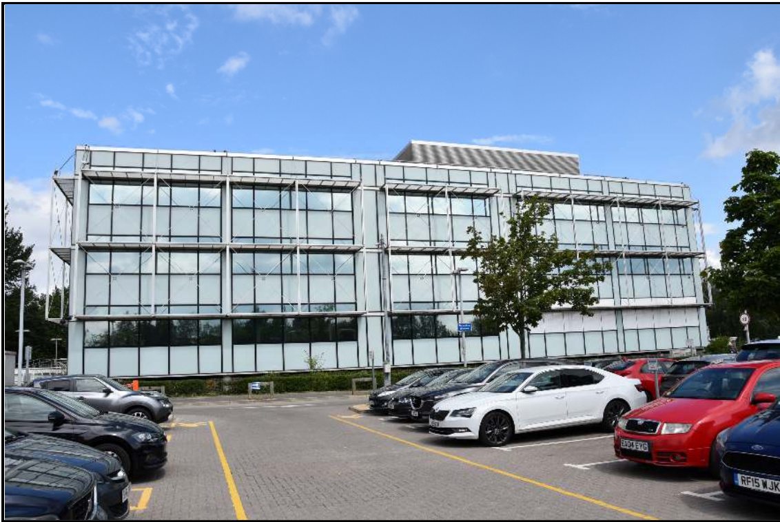
Plate 3 Southern elevation and car park
