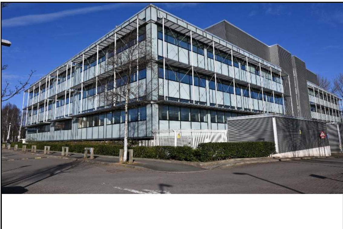
Plate 2 Building 2 Southern and Eastern Elevation
