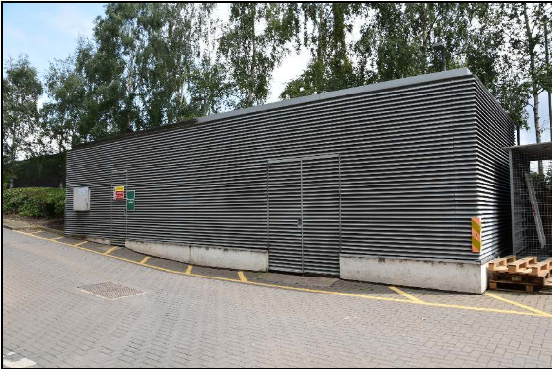
Plate 5 Oil tank housing 2No 6500 litre tanks
