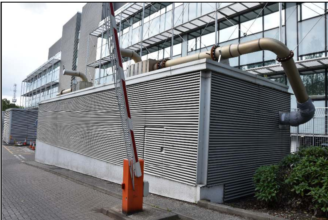
Plate 4 Generator house outside the eastern elevation
