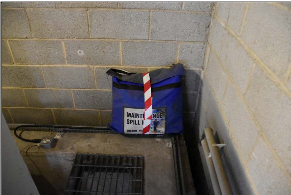
Plate 10 Spill kit in tank area
