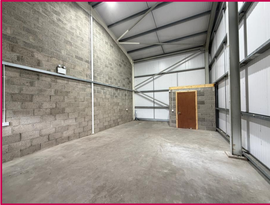
Ample space for mezzanine floor if desired
