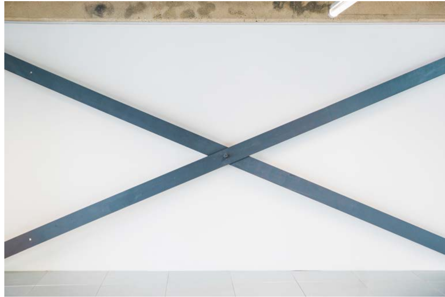
Retained heritage feature on floor 2
