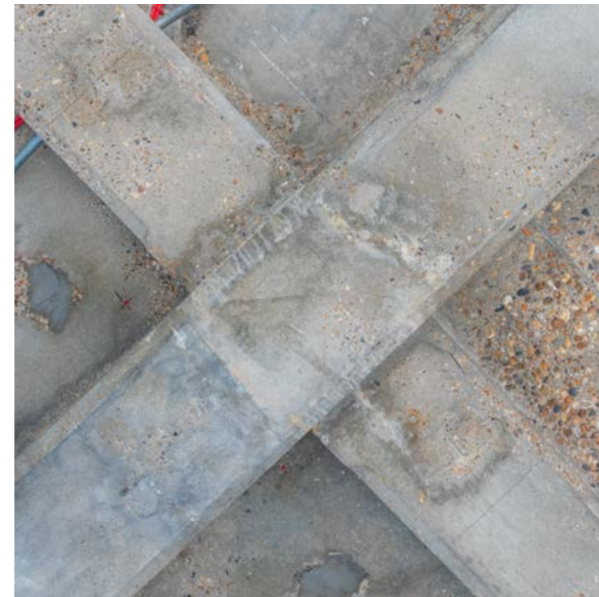
Exposed concrete feature
