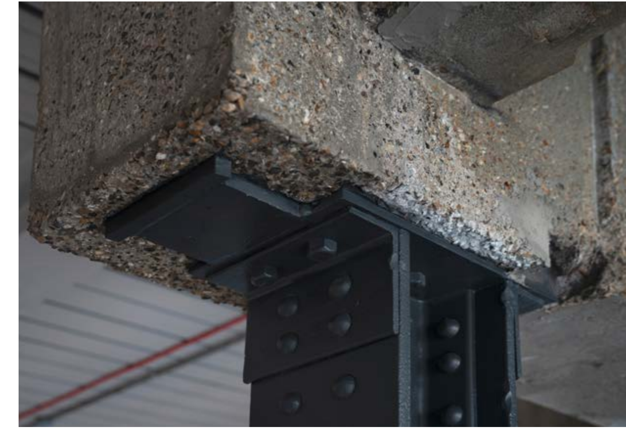
Retained heritage concrete knuckle
