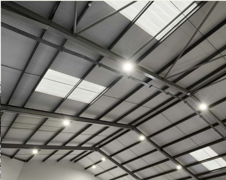
● Newly fitted roof panels for enhanced natural lighting increasing staff welfare and efficiency
