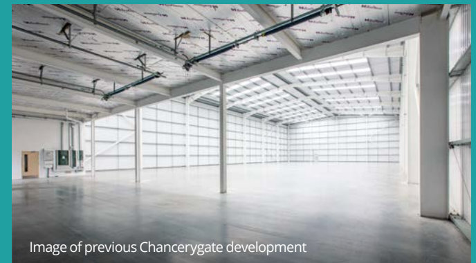
Image of previous Chancerygate development
