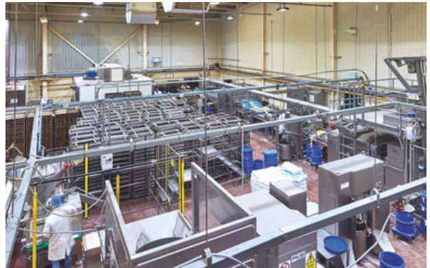
Unit interior prior to refurbishment
