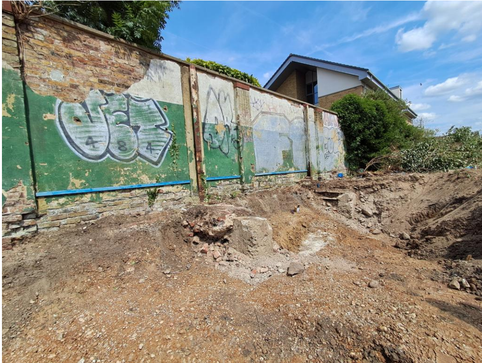
Installation of Root barrier membrane
