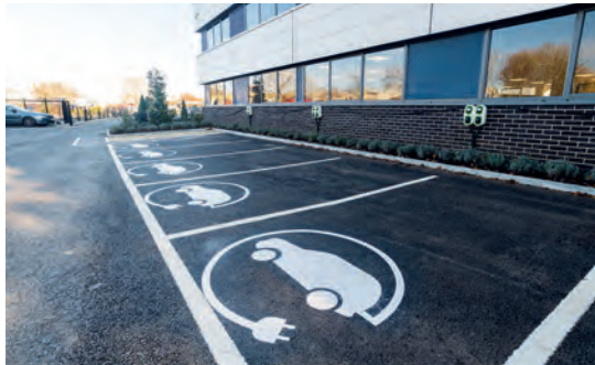
Westerly elevation showing electric vehicle charging points
