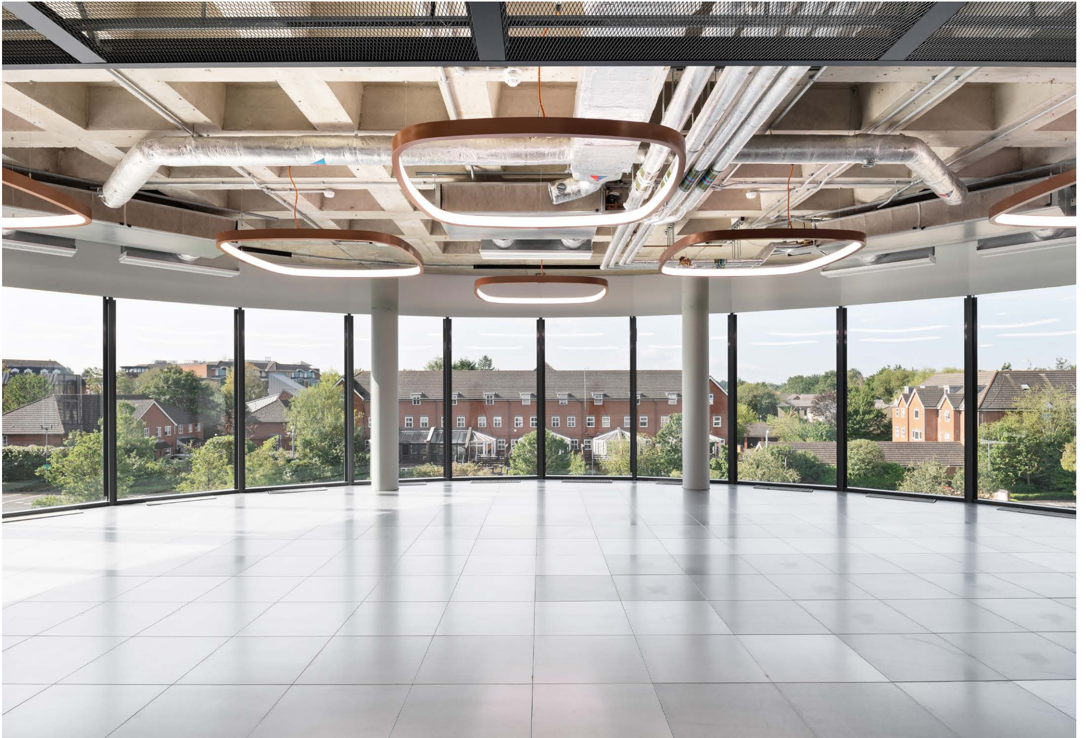
SECOND FLOOR OFFICE
