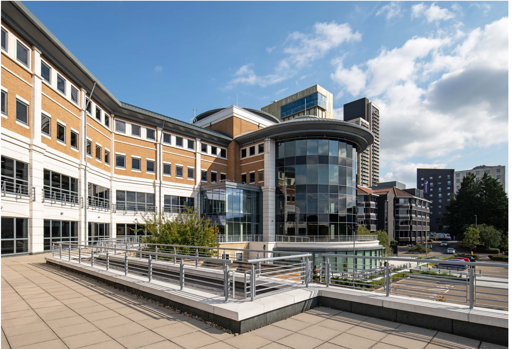
FIRST FLOOR ROOF TERRACES
