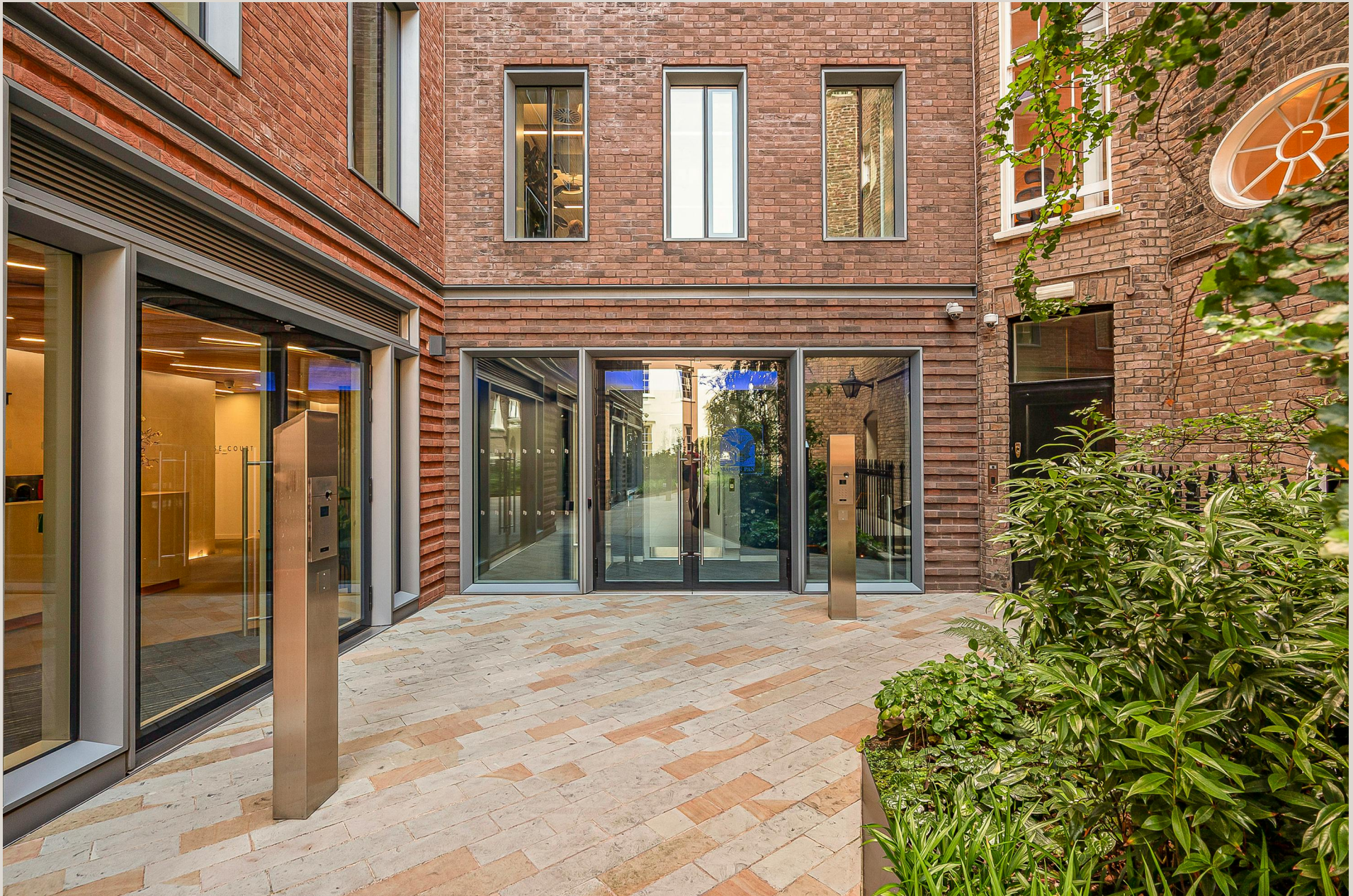
The Vaults - Hobhouse Court, 3-5 Whitcomb Street
