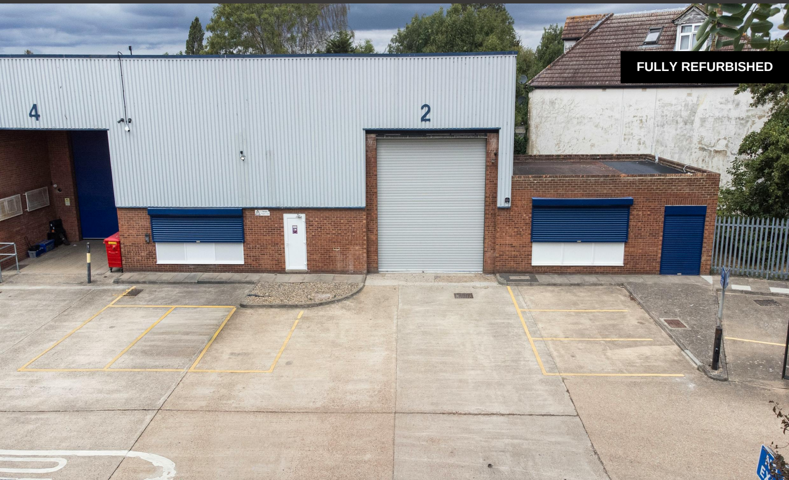
Unit 2, Barratt Way Industrial Estate Barratt Way, Harrow, HA3 5TJ
